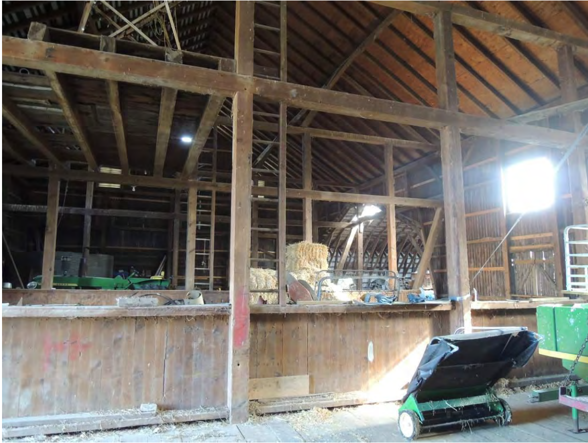
Photo 28: Barn Complex, original Barn, Upper Level. View facing E through framing. Note the gambrel tresses of the addition roof at rear right of view.
