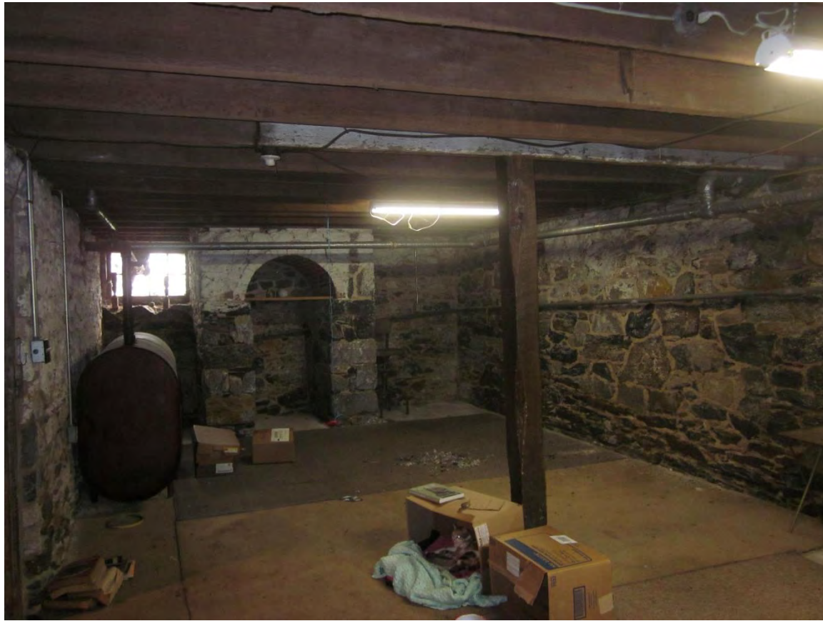
Photo 20: Mifflin House, Cellar, South Room, view across room facing E. Note arch supporting chimney stack, typical at each end of this room.
